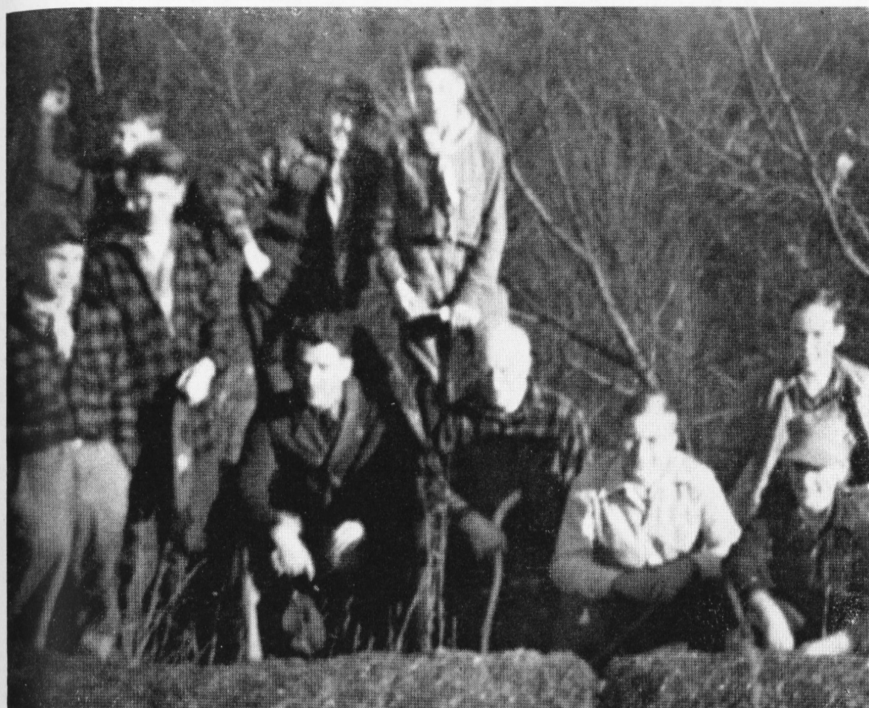
Above is George Rowell's Scout Troop II of Watertown and their guest for the day, Arthur P. Hickcox. The boys and George have been busy on Sundays of late starting the building of new trails in Black Rock Park. Immediately beneath the group, in the rear of the rock upon which they are standing, is the well known "Leatherman's Cave."
